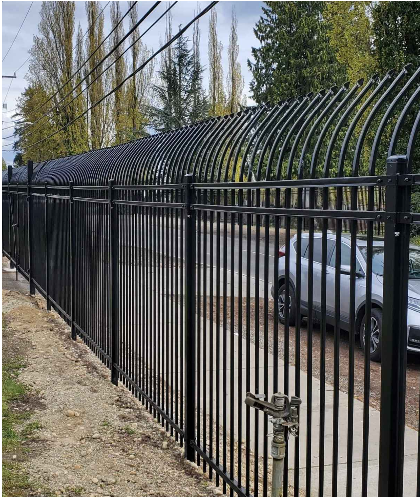
EXAMPLE PERIMETER/SECURITY FENCE
