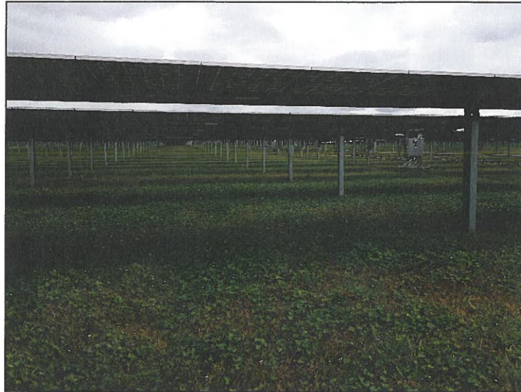
Figure 3 - Established vegetative cover at an operational solar facility built by Strata in Virginia
